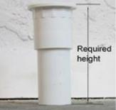
Cut pipe from floor and connect hub. Required height is from Step 1. Apply some caulk to the top flange of the hub to hold the silicon gasket in place. Lift tub over drain.
