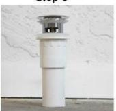
Seal the top of the drain basket as noted above. Unscrew pop-up and use a basket wrench to tighten the drain basket into the hub. Allow to dry and then re-attach the pop-up, fill with water and test for leaks
