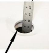
Measure height from floor to this point under the bathtub drain hole. This will determine the height from
